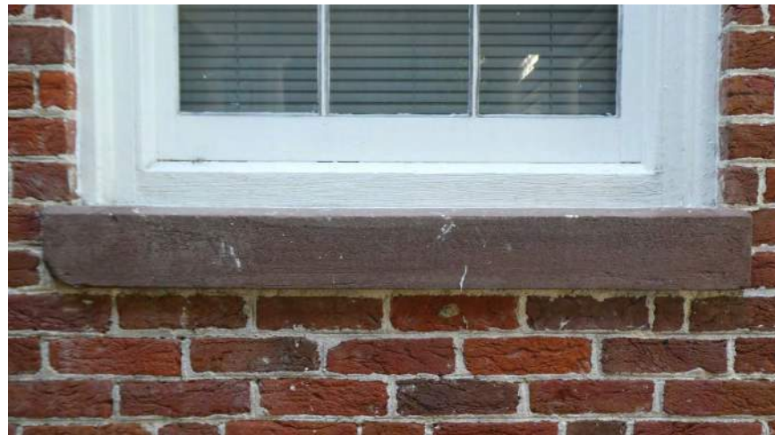
Precast Sills and Bands Match Existing
